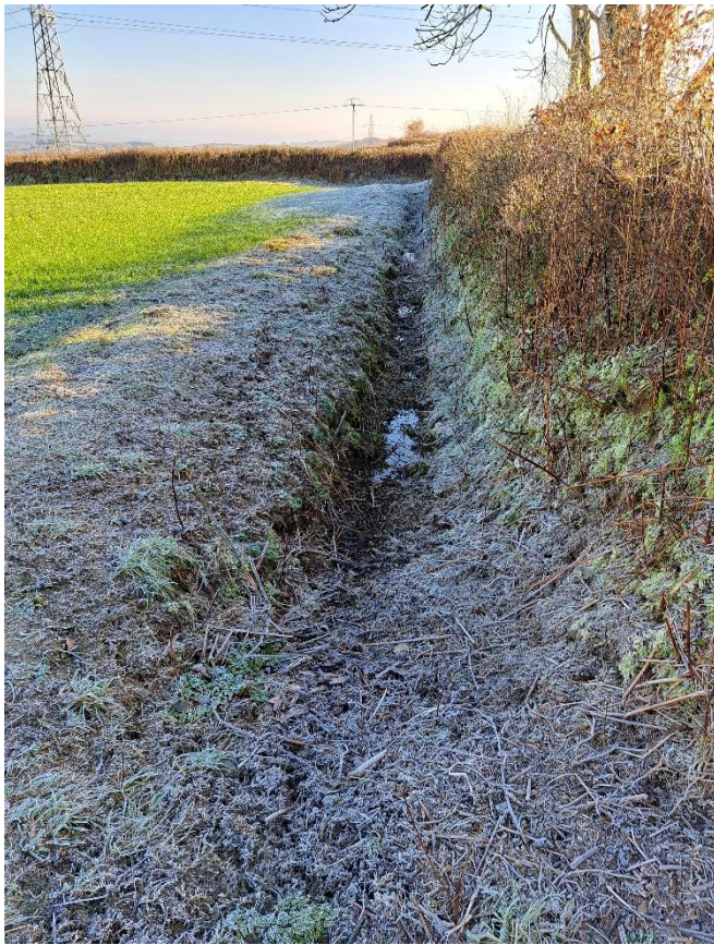
Plate 14: Area 1 – South Boundary Ditch (E)
